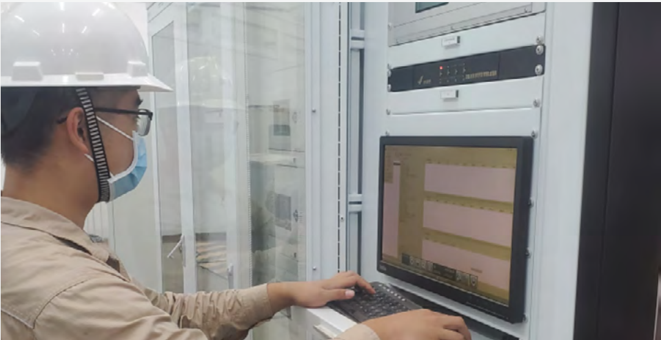
A commissioning engineer of NARI is conducting synchrophasor measurement and commissioning
