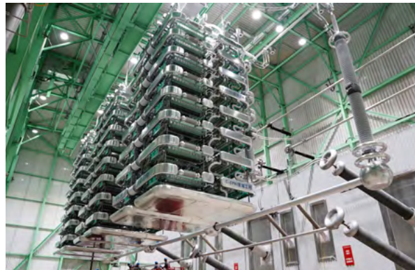
The site of the CLCC converter valve at Shanghai Nanqiao Converter Station
