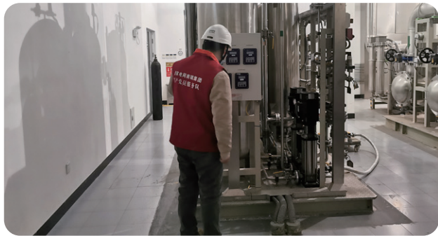
Routine inspection on the water-cooling system of the converter valve
